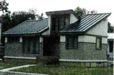
Solar Homes under construction
